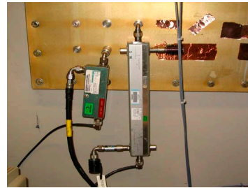
FIGURE 11B - SCREEN ROOM ACCESS PANEL WITH DIRECTIONAL COUPLERS
