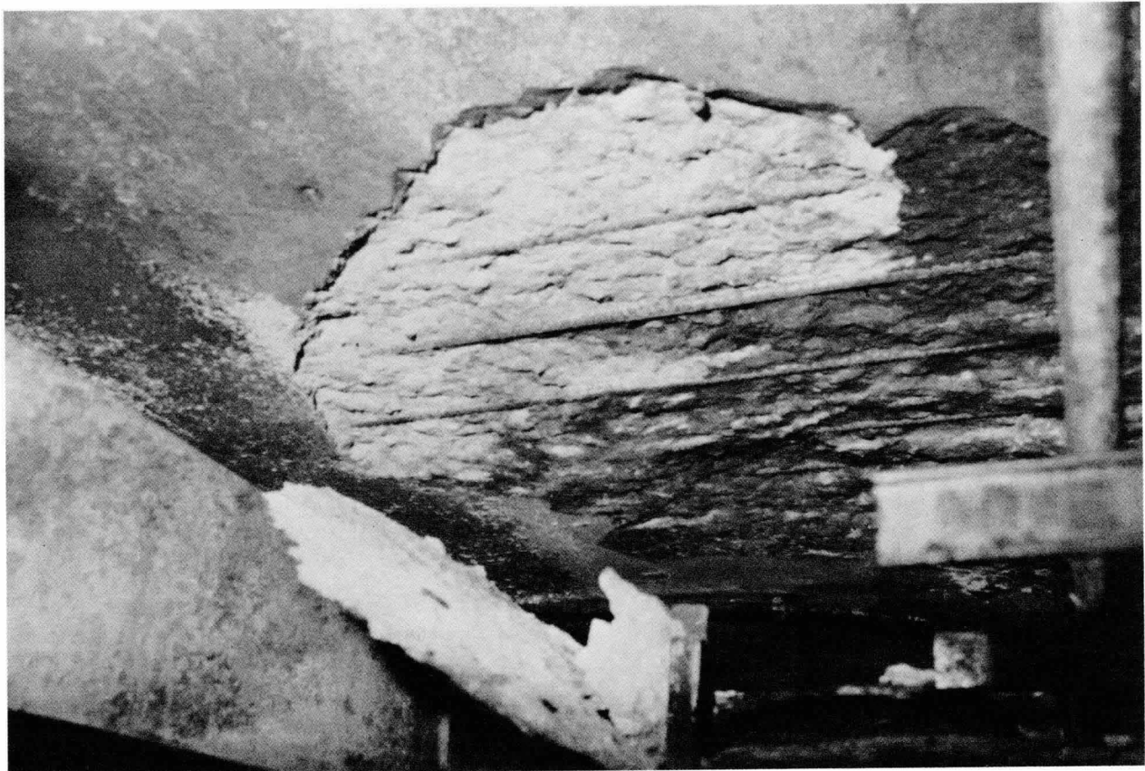
Figure 4-6 Spalling on ceiling.
