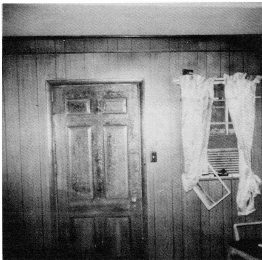
Figure 4-19.2 Blistering of varnish on door and slight scorching of draperies are the only indications of the natural gas flash fire.
