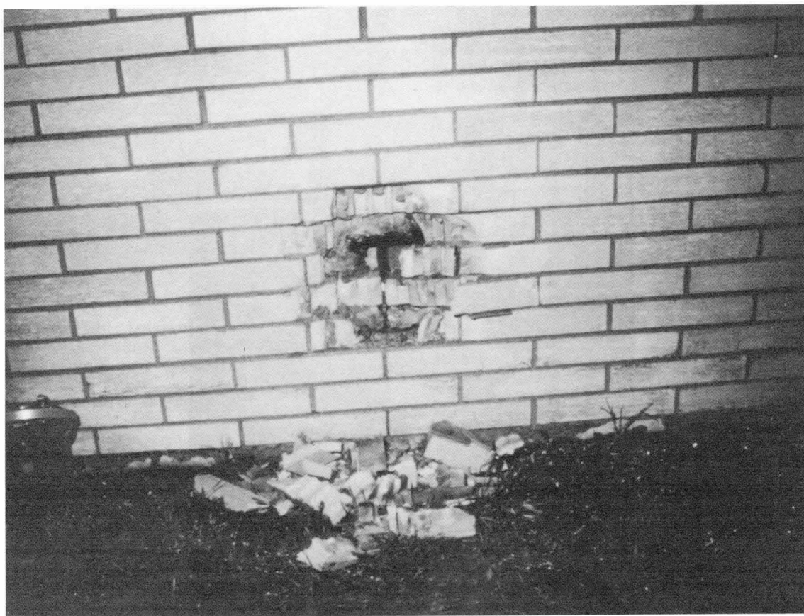
Figure 4-20.2 Damage to an outside brick wall caused by thermal expansion of an I-beam in the basement.
