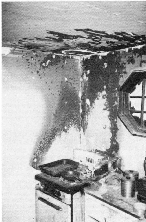
Figure 4-11 Clean burn on wall surface.
