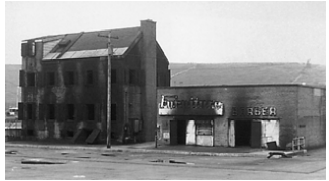
Figure 7-9 Both flat and sloped roofs can be designed into a burn building. (Courtesy of Nassau County Fire Training Academy, Old Bethpage, NY.)
