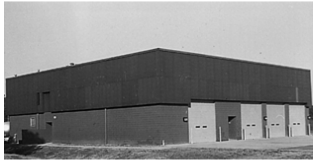
Figure 10-1.2(a) Fire apparatus building, housing classroom. This building is approximately 100 ft (29.9 m) long with five 15-ft (4.5-m) overhead doors, classroom, maintenance area, and apparatus storage area. (Courtesy of Mississippi Fire Academy, Jackson, MS.)
