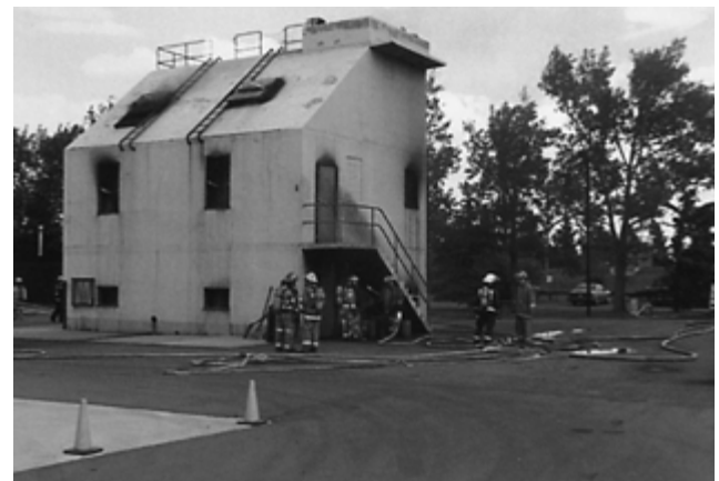
Figure 8-1(b) Burn building with provisions for basement fires and roof ventilation. (Courtesy of Alberta Fire School, Edmonton, Alberta, Canada.)
