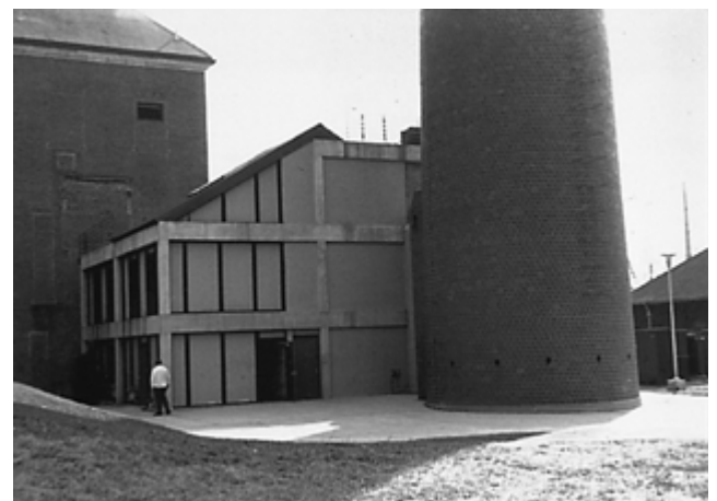
Figure 10-1(b) Combination building—maximum use of minimum space with existing smoke stack for EPA considerations. This building provides for ventilation, smoke chamber, rappelling, laddering, live fire training, sprinkler laboratory, gas and electric cutoff, and forcible entry.
