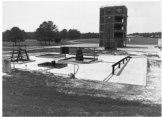
Figure 11-2.3(c) Portable fire extinguisher training area. Training area is 75 ft × 85 ft (23 m × 26 m). Seven training scenario areas are located on this pad. (Courtesy of Mississippi Fire Academy, Jackson, MS.)
