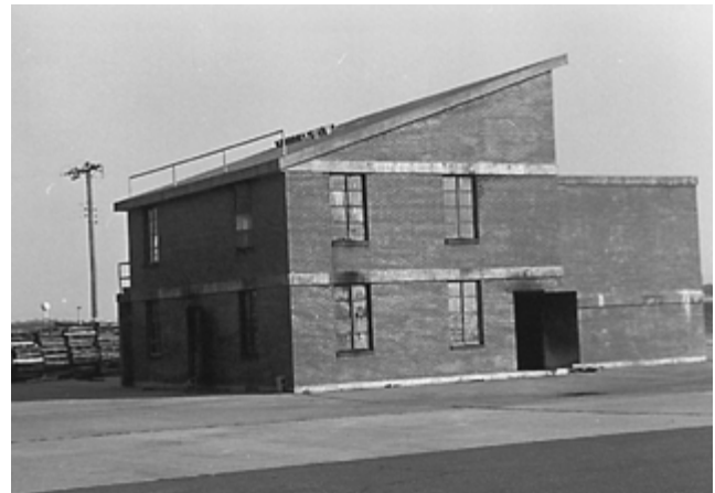
Figure 8-1(a) Hot drill building. This building features two buildings in one—residential and commercial. The residential side is two stories with attic and six interior rooms, all masonry. (Courtesy of Mississippi Fire Academy, Jackson, MS.)
