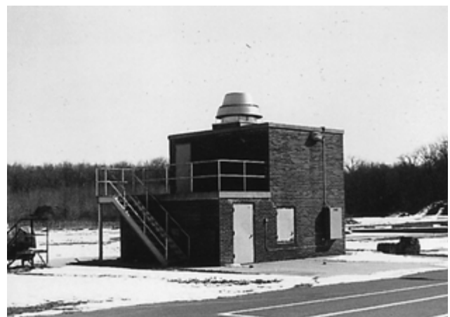
Figure 9-1.1 Smoke building with exhaust fan at roof level. (Courtesy of Burlington County Fire Academy, Burlington County, NJ.)
