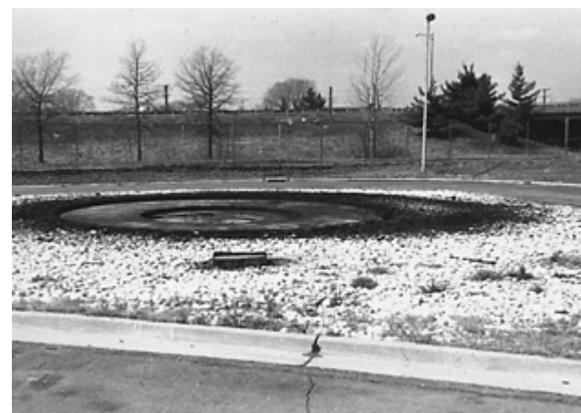
Figure 11-2.2 District of Columbia Fire Department flammable liquid pond. Note the heavy stone surrounding pond. (Courtesy of District of Columbia Fire Department, Washington, DC.)
