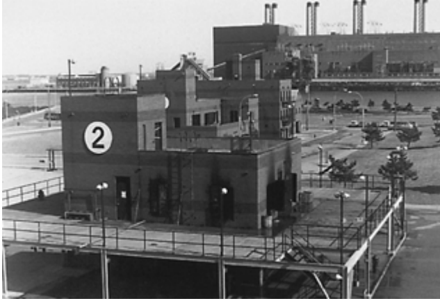
Figure 8-1.1 Burn building with raised open-grid walkways level with the second floor. (Courtesy of New York Fire Department Fire Academy, New York, NY.)
