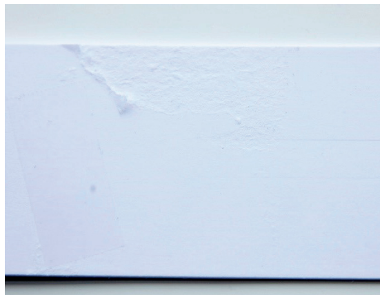
Figure B.4 — Damaged surface, e.g. from adhesive tape
