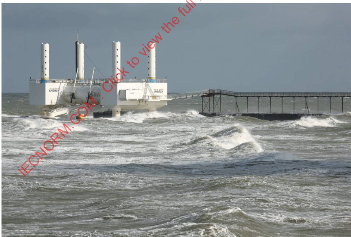
Figure F.1 – The Wavestar prototype (diameter of each float is 5 m)
